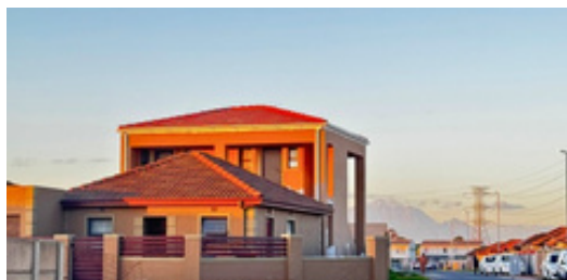
4 bachelor units in Eersterivier completed in 2025 (Photo: Anika Hanekom, 2025)
