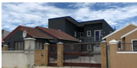
6 bachelor units in iLitha Park completed in 2022 (Photo: Vunene Xiluvane, 2024)
