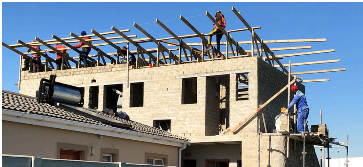
Construction team installing the rafters for a roof for a 4 rental unit flats in the backyard of a home in Eersterivier, Cape Town (Anika Hanekom, 2023)
