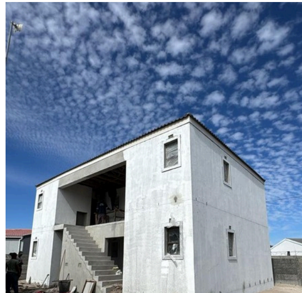
An 6-unit bachelor unit under construction in Mandaly (Photo: Anikam Hanekom, 2026)
