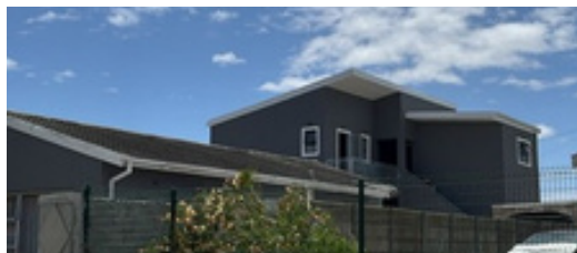
6 bachelor units in Mandalay completed in 2026 (Photo: Anika Hanekom, 2026)
