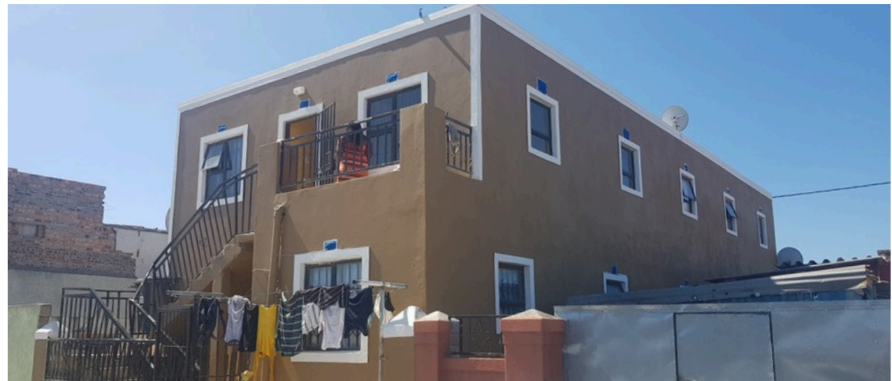
18 Flats built in 2019 using a homeloan from iBuild (Photo: Connie Guda, 2021)
