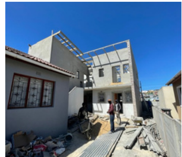
Rental units under construction in iLitha Park (Photo: Abongile Mvukuzo, 2022)
